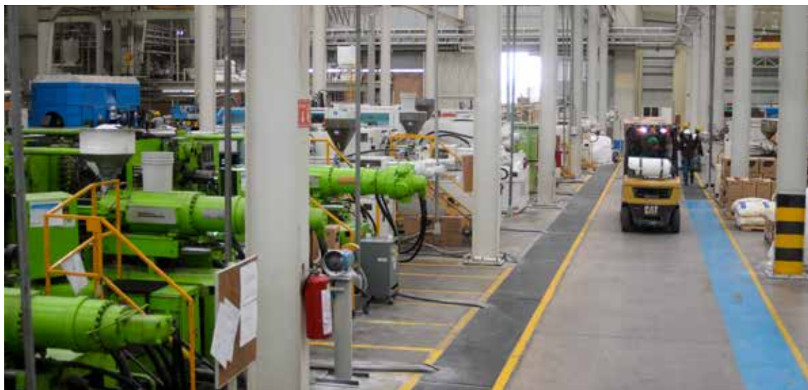
PVC pipe process, Colombia
