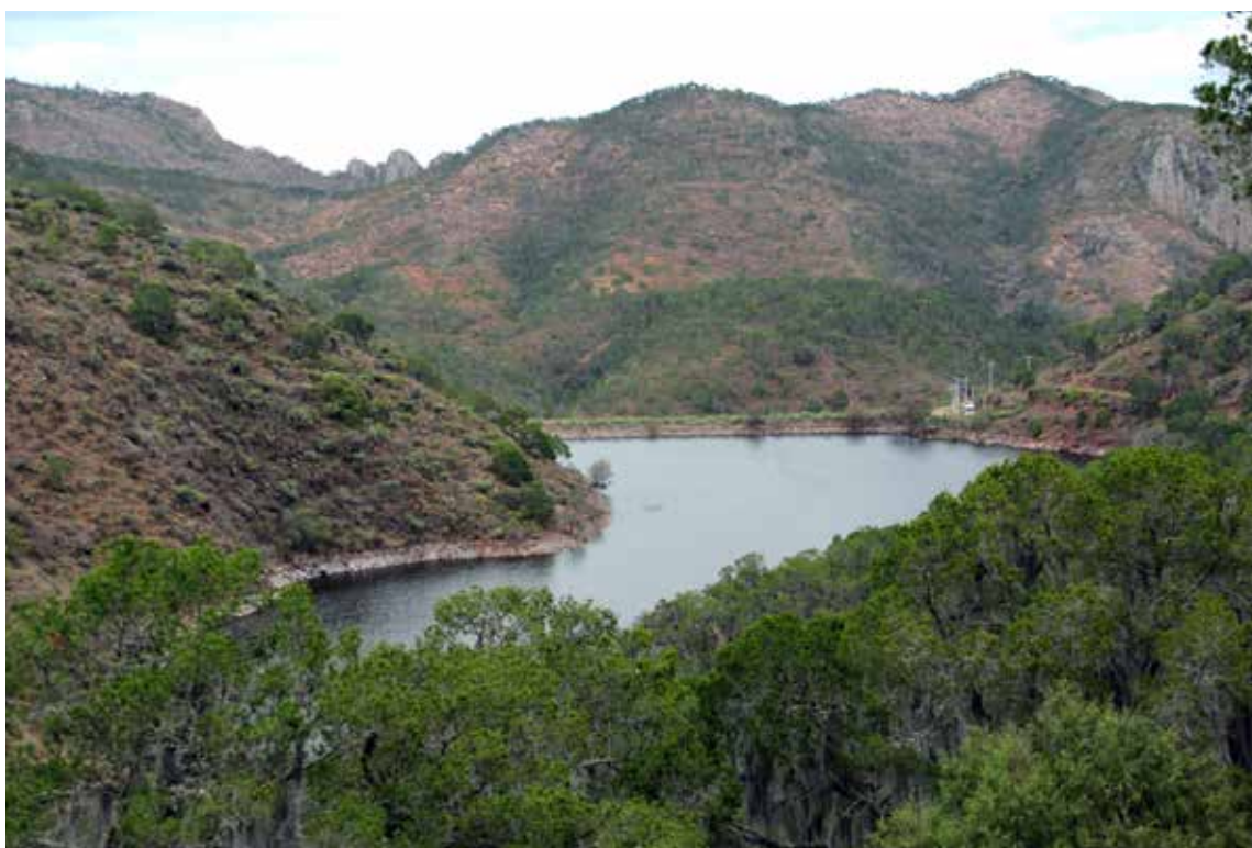
Water dam, fluorite mine in San Luis Potosí, México
